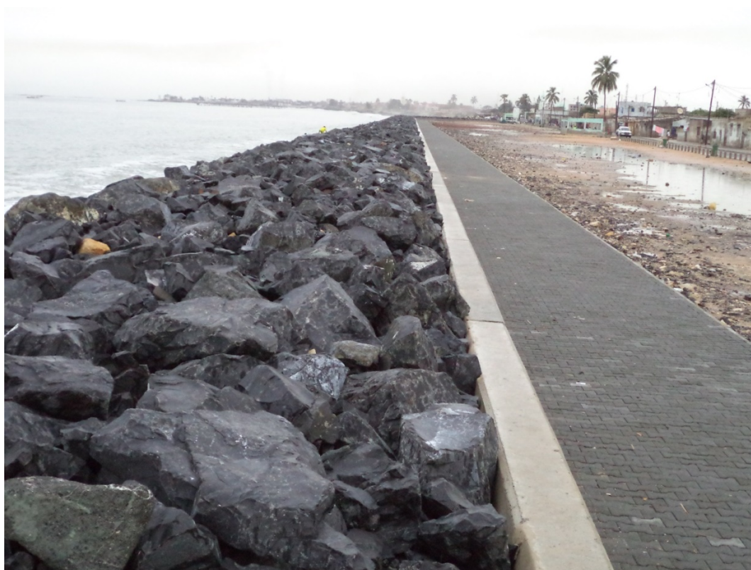
Photo 4: Seawall protecting the houses (Saly)
